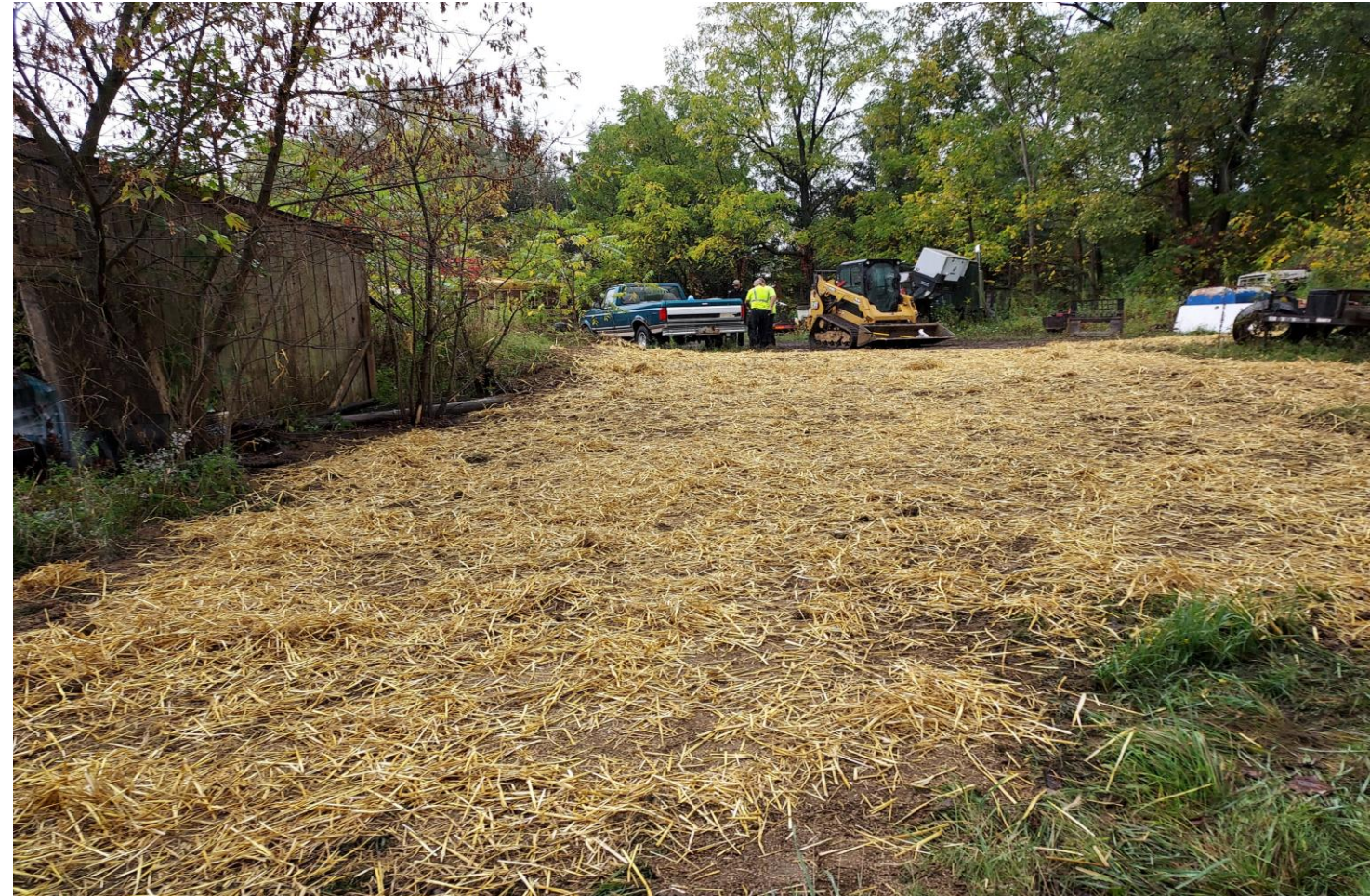
Photo of site after remediation
