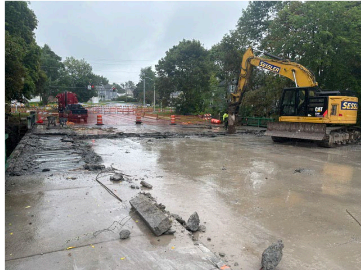
Beginning deck removal
