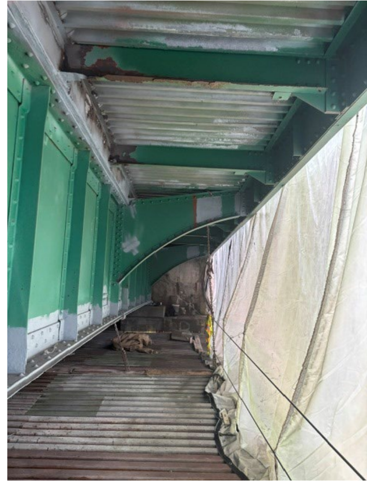
Localized cleaning and painting of bridge, primer coat shown.
