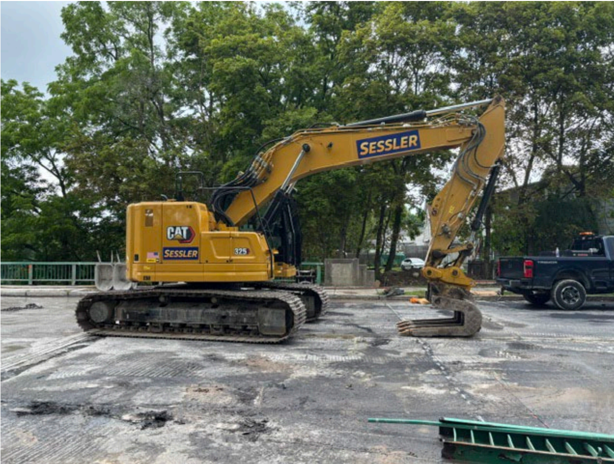
“Slab Grabber” bucket mounted to an excavator to be used to remove the bridge deck,
