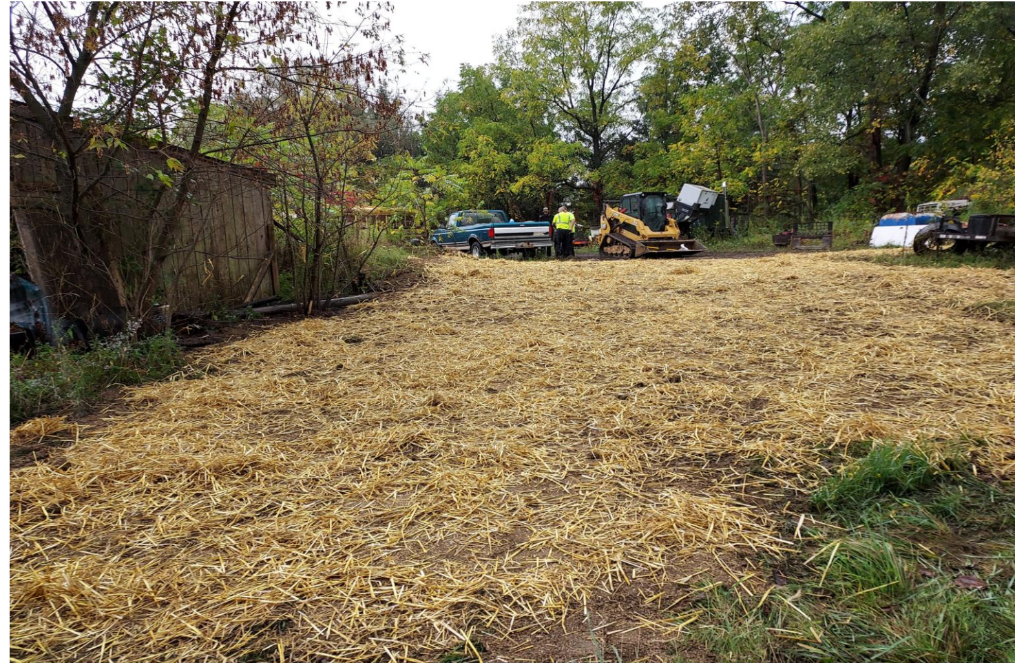
Photo of site after remediation
